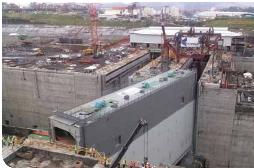
In another major milestone for the Panama Canal Expansion Program, the electro-mechanical installation phase, one of the most important of the project, has begun with the installation steel rolling gates. All gates are to be installed by mid-2015. Photo credit: Panama Canal Authority.
